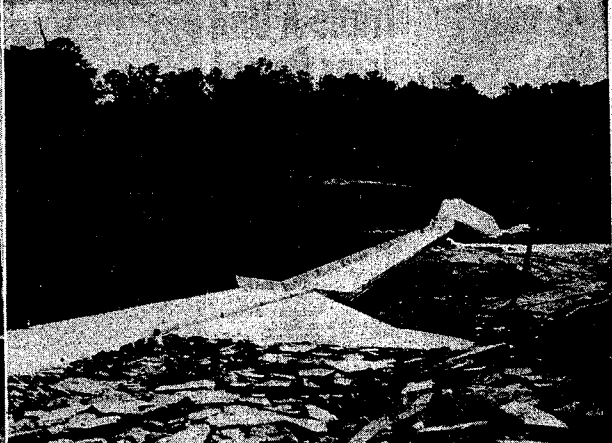
of the Infantry School, cuts the tape, officially opening the dam. The right photo shows a view of the dam. Its purpose is to supply a deep enough pond to allow for river crossings since the Chattahoochee river, according to engineers, is too swift and unpredictable, especially during the flood season.
